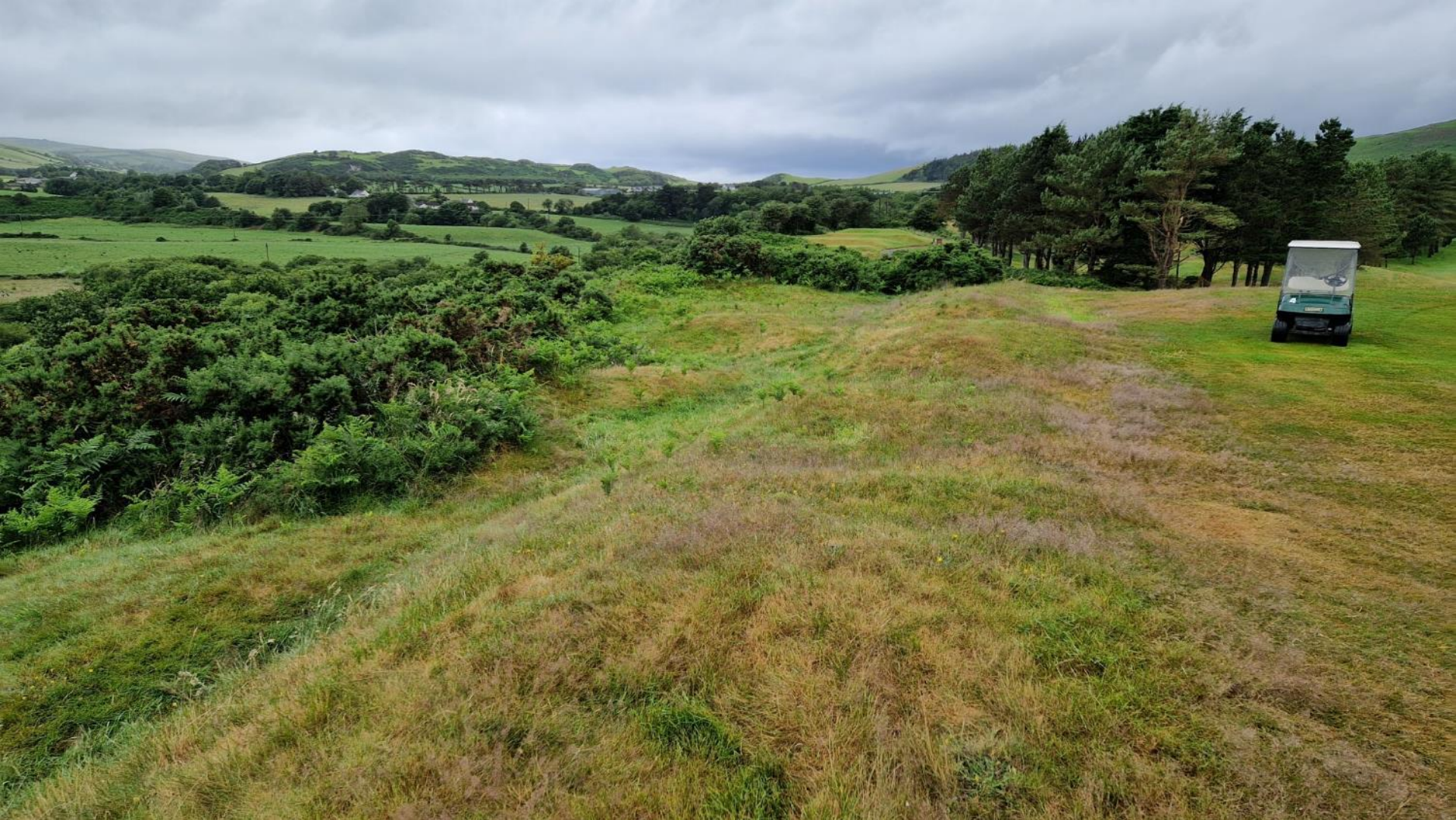
Gorse removal & earth-shaping to create new fairway
