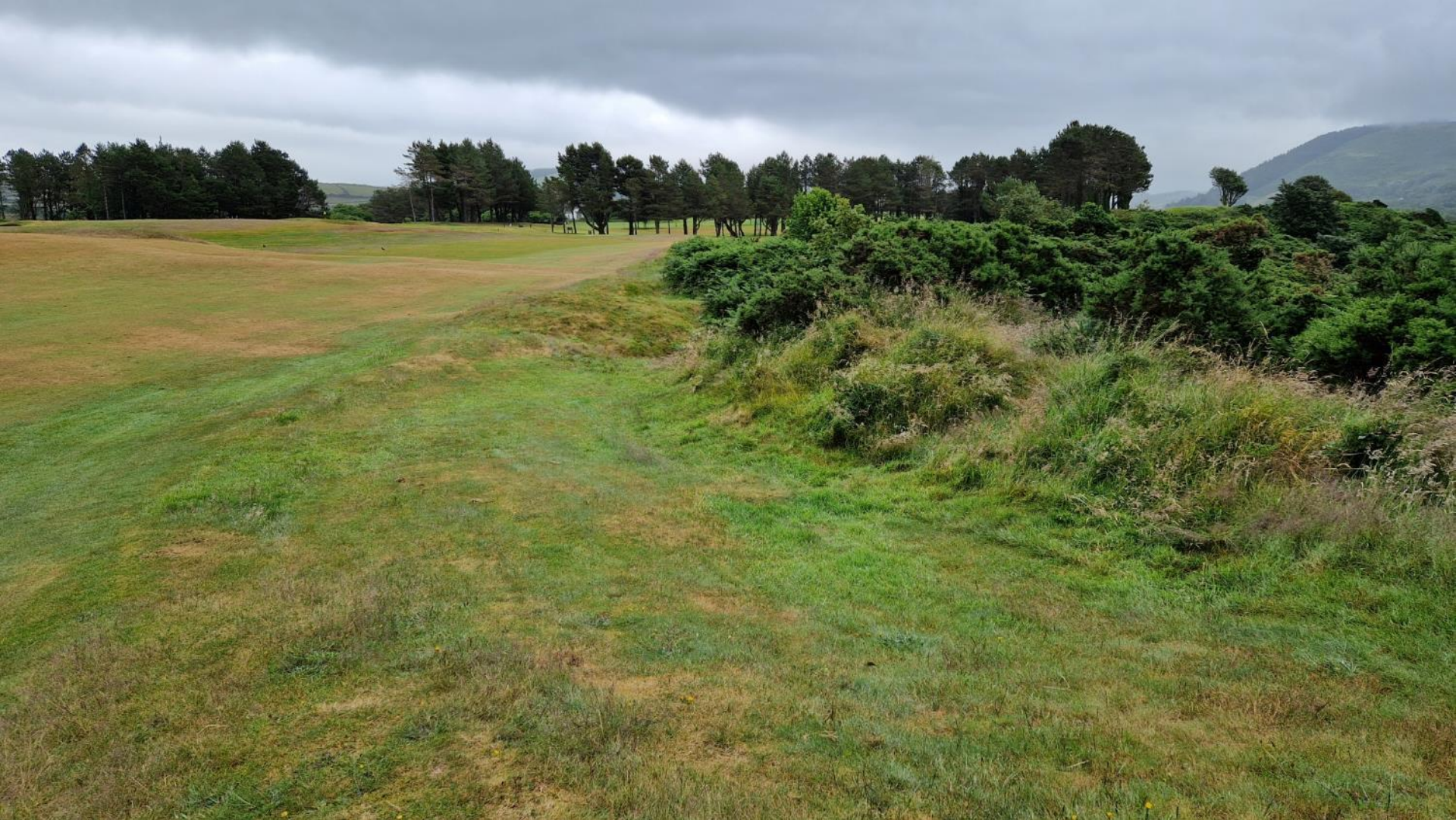
Gorse removal & earth-shaping to create new fairway
